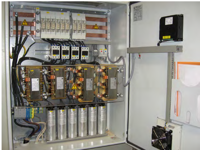
Figure 14: Example of a power factor correction unit used for plant-wide power factor correction. Notice the bank of capacitors located at the bottom of the unit.
