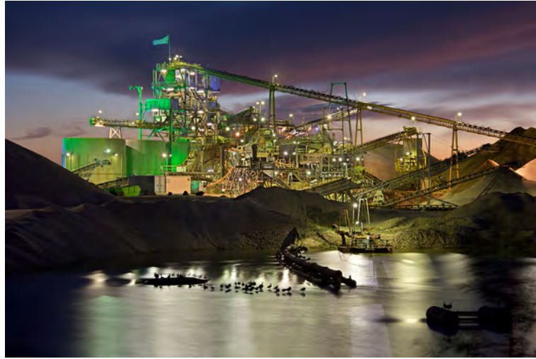
Figure 3: Large industrial plants containing motors and other reactive loads in constant or near constant operation (such as the large conveyors in the mining plant in the above figure) greatly benefit from power factor correction.
